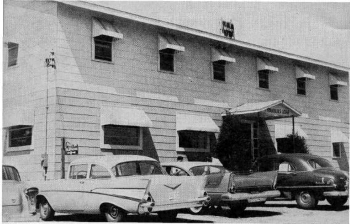
Hotel facilities, Franklin's Lodge, Lake Ivanhoe
