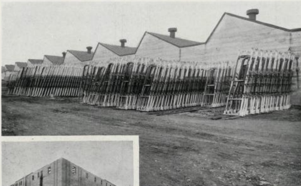
Exterior View of Frame Dept.
