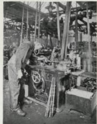
Grinding Cam Shafts
