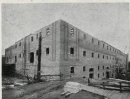
Warehouse in Construction
