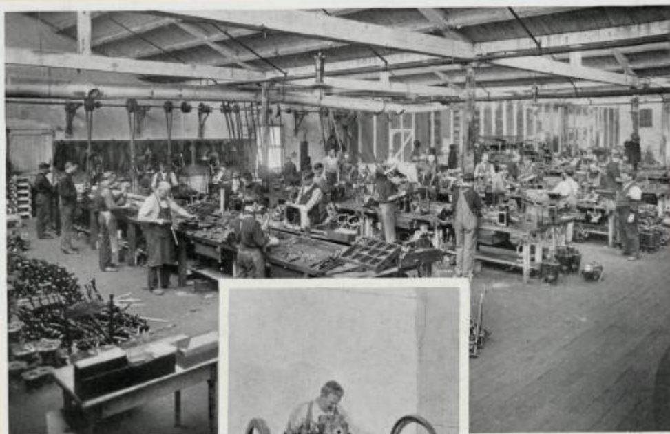
Transmission Assembling Room
