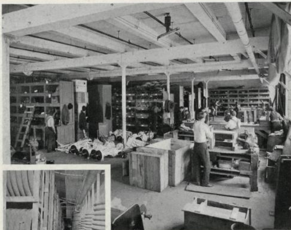
Repair Parts Stock Room
