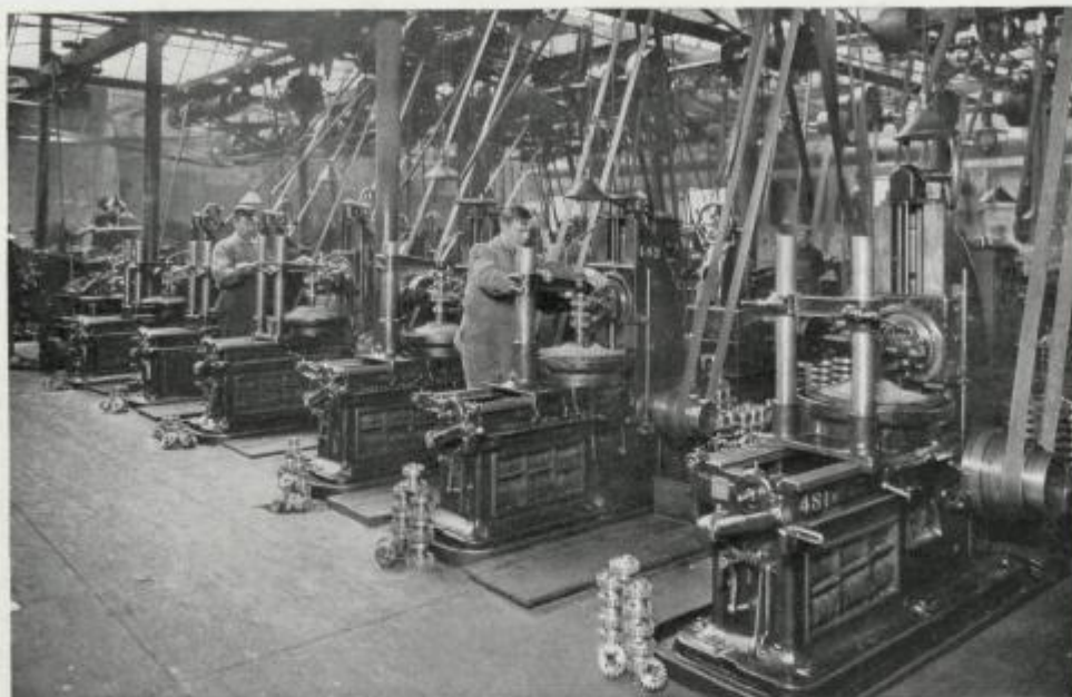
Gear Cutting Machines
