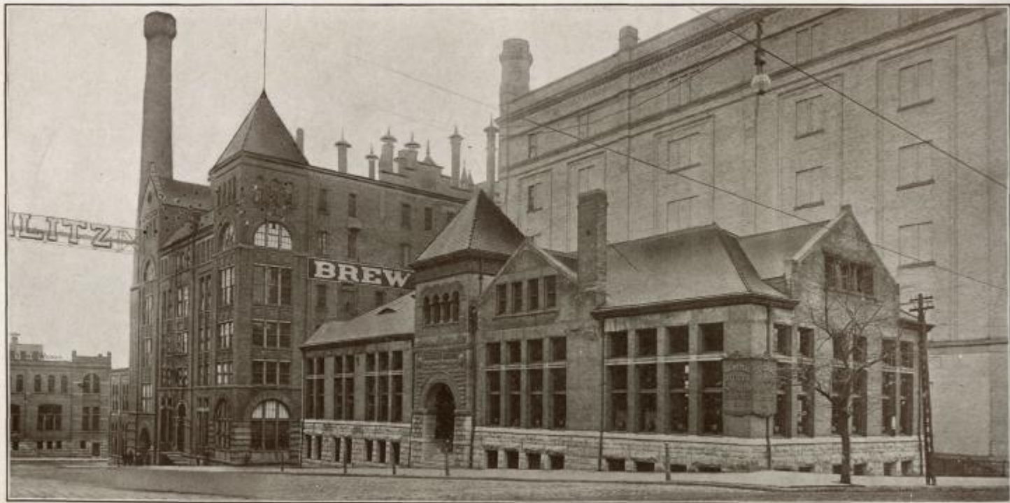
GENERAL OFFICES Brew House and Bottling Department in Background
