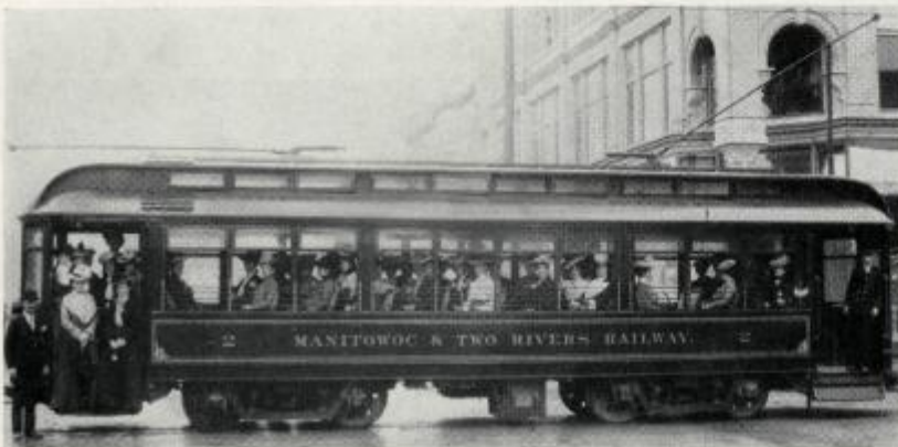
The old inter-urban line between Manitowoc and Two Rivers was the principal means of transportation between the two cities. Mr. Thomas Higgins started the line in 1902.
