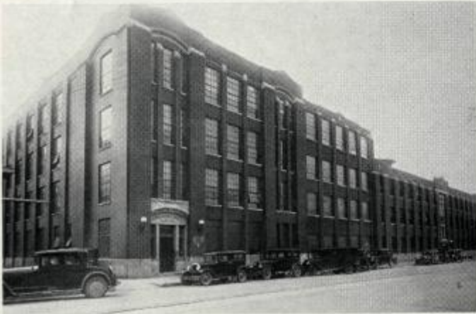
This portion of Plant 1, facing 16th street in Two Rivers was built in 1919.
