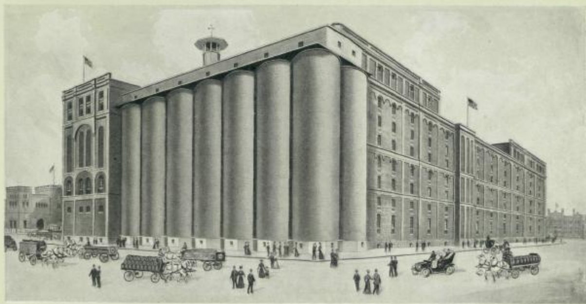
THE GLAZED TILE CIRCULAR MALT STORAGE ELEVATOR
