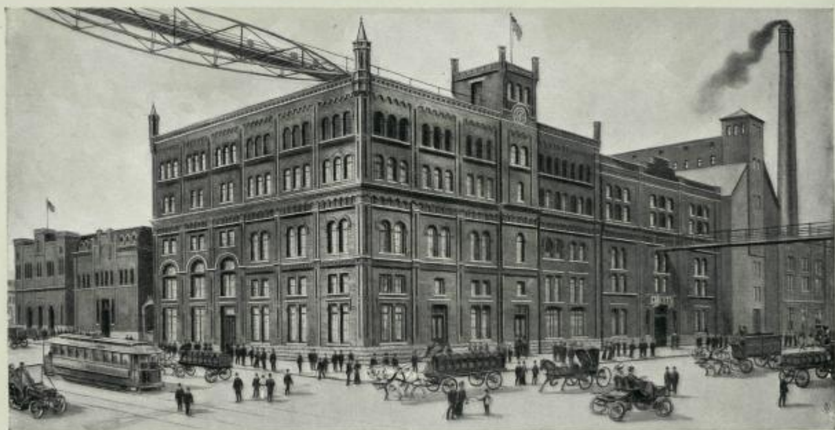
MACHINE HOUSE, ELECTRICAL POWER HOUSE, REFRIGERATING PLANT
