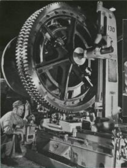
(Above) Hobbing 2 helical gears for Speedcrane transmission
