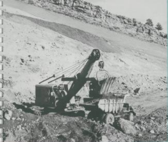
Model 350 manual shovel at work on the new Dams project in Colombia.
