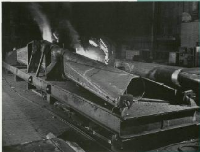
Held rigidly in place in a jig to prevent distortion, a steel beam is being welded together.
