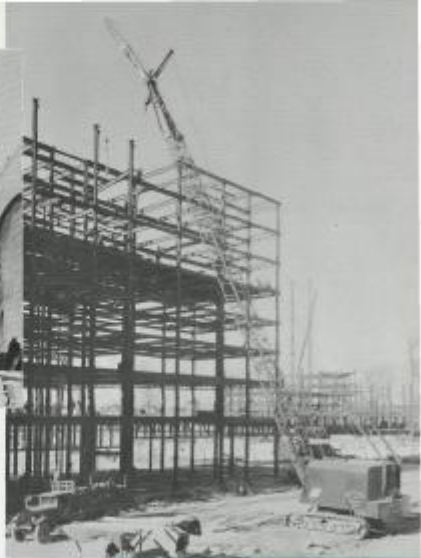
(Right) A Manitowoc Speedcrane with 100-foot boom and 30-ton jib shown setting steel on a building.
