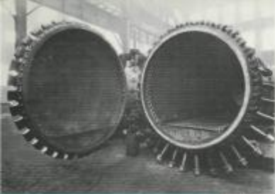
(Left) The open ends of a rotating cylinder used for testing rollers.
