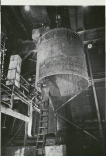
(Right) Fitting longitudinal beams on a boiler shell.
