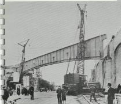
(Above) Two Model 900 Speedcranes place a girder (137 feet long; weight 185 tons) on its supports at the New Jersey entrance to the Lincoln Tunnel.
