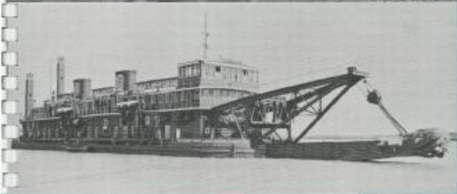
Bully in 1927 for the Great Lakes Dredge & Dock Co. of Chicago, the Muck Dred Electric Hydraulic Dredge NEW HESLEY is one of the largest, most powerful dredges of this type on the Great Lakes.
