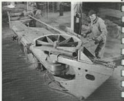
(Above) Bending 6-inch pipe by machine.
