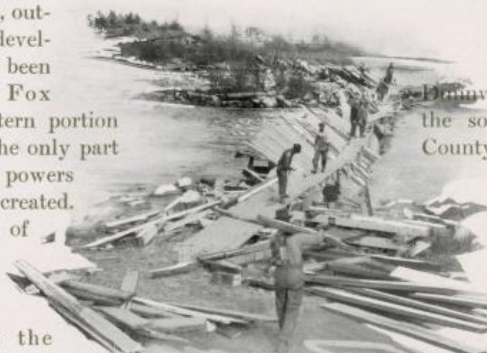
Making the First Coffee-Dam
