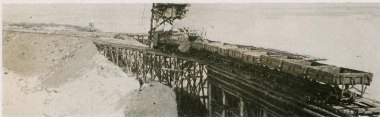
Making Earth Fill at North End of Dam
