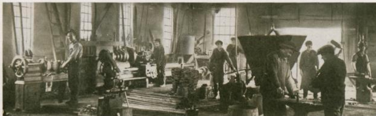
Interior of Blacksmith and Machine Shop
