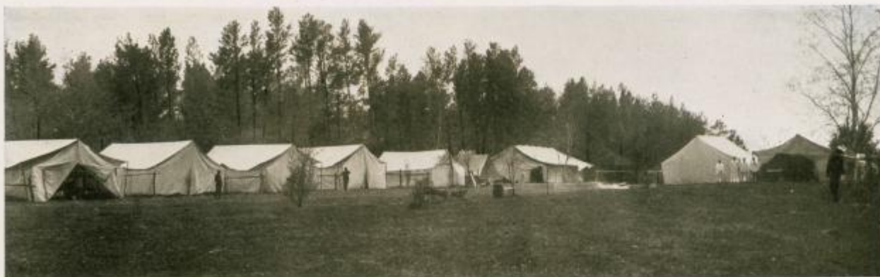
Transmission Line Builders' Camp
