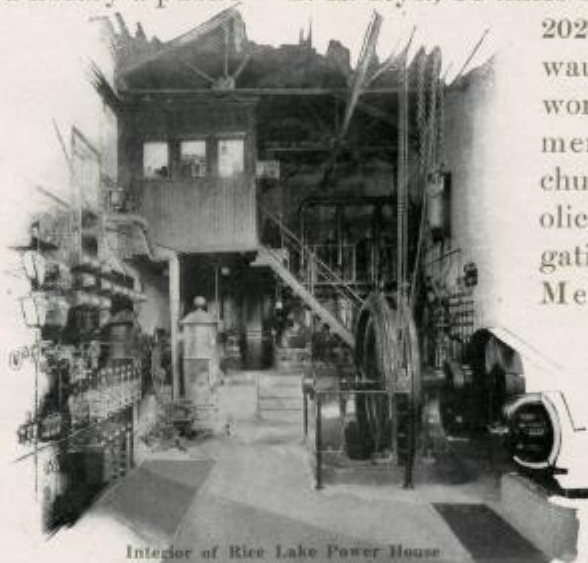
Interior of Rice Lake Power House
