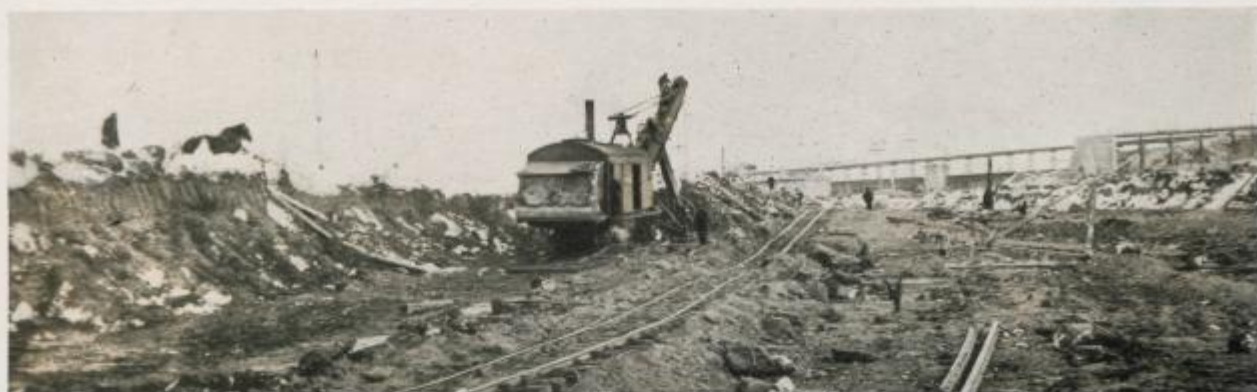
Work of the Steam Shovel
