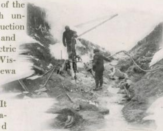
Testing the River Bottom for Foundations
