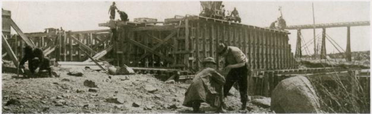
Locating Center Line of Buttresses
