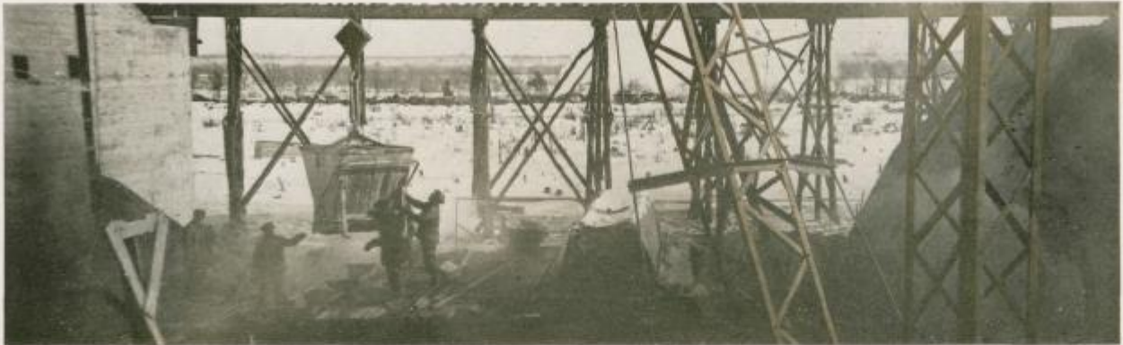
Pouring Concrete in Abutment
