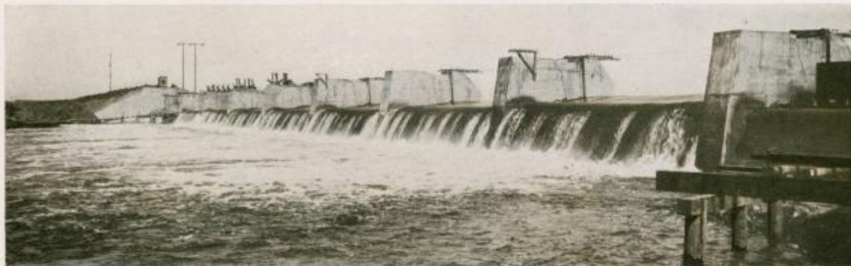
Water Running Over Spillway
