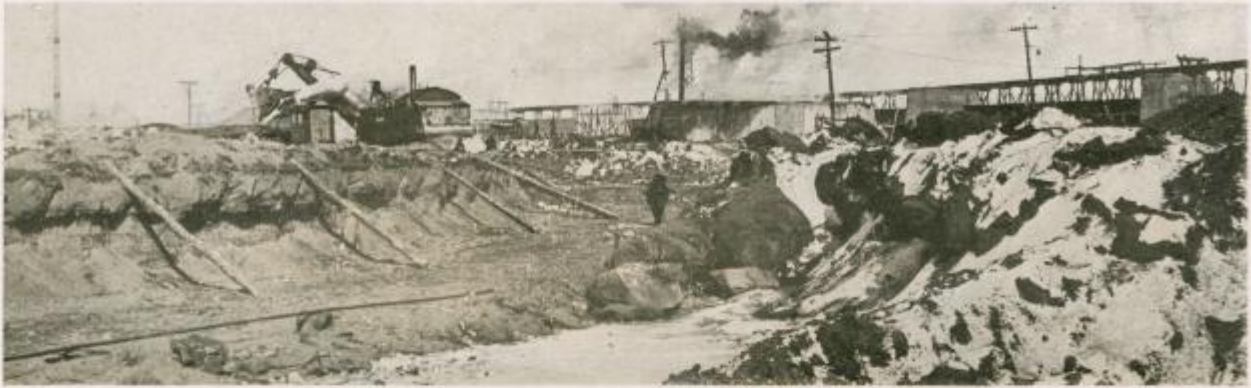
Excavating in Spillway Channel
