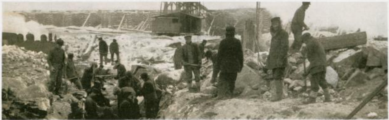
Excavating for Power House
