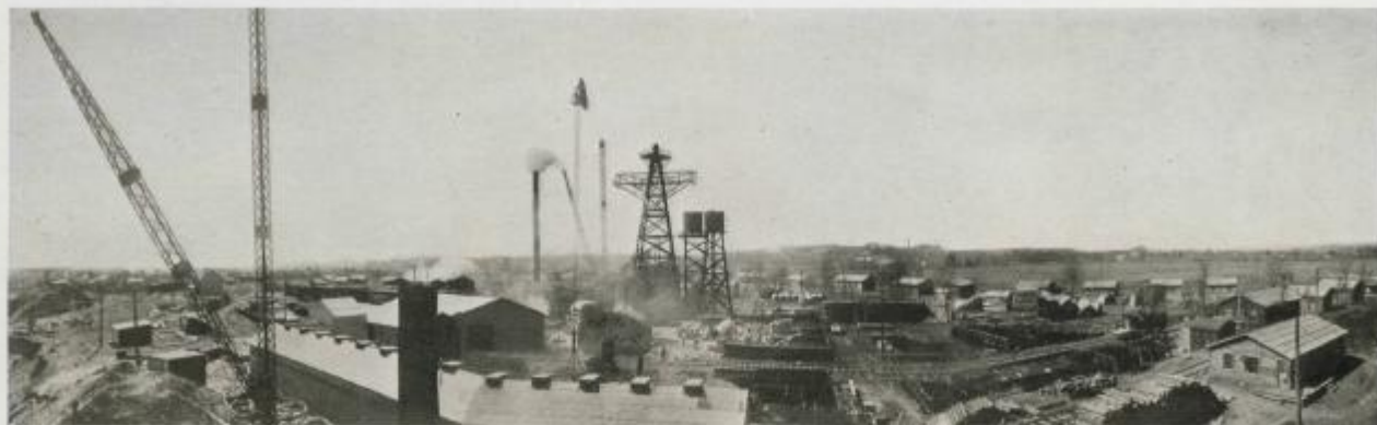
Panorama View of Construction Works at the Dam
