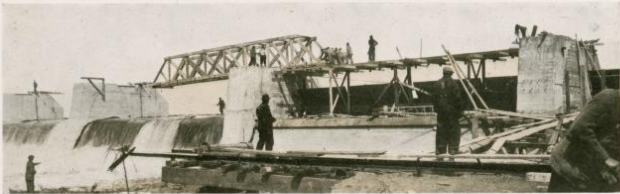
Another Stage of Flood-Gate Setting
