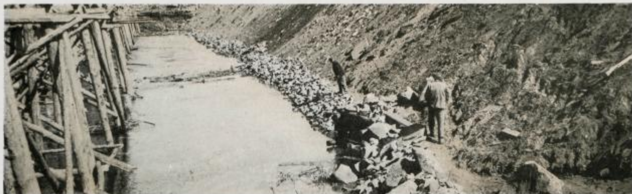
The Earth Dam Growing
