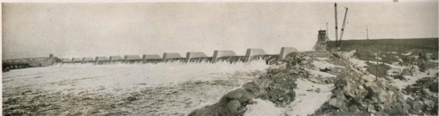
Down Stream View of Wisconsin Dam
