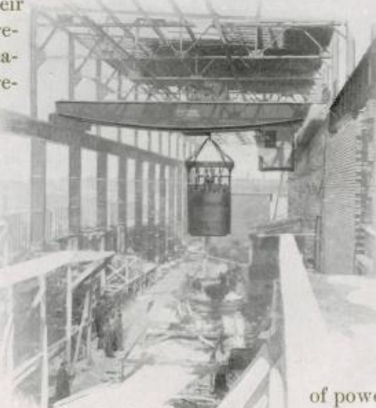
Placing Transformer Weighs 21 Tons
