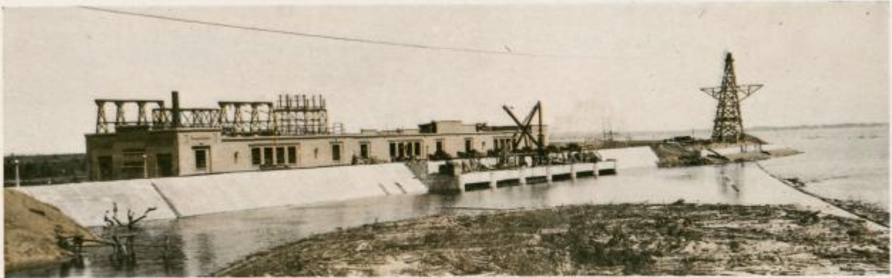
Up-Stream View of Power Station
