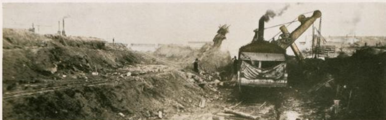
Tearing Out the Rock of the River Bed
