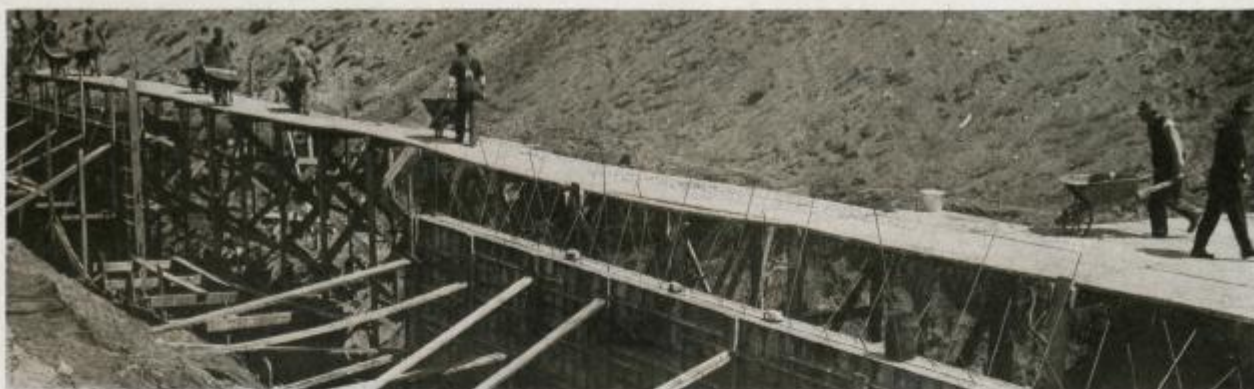
Pouring Concrete in Corewell
