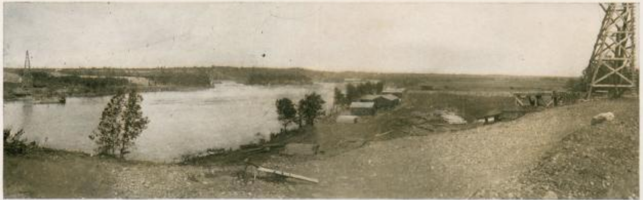
Bringing in Construction Material
