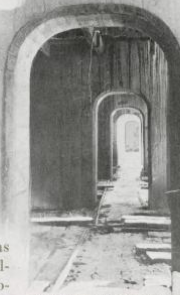
Runway through Hollow Dam
