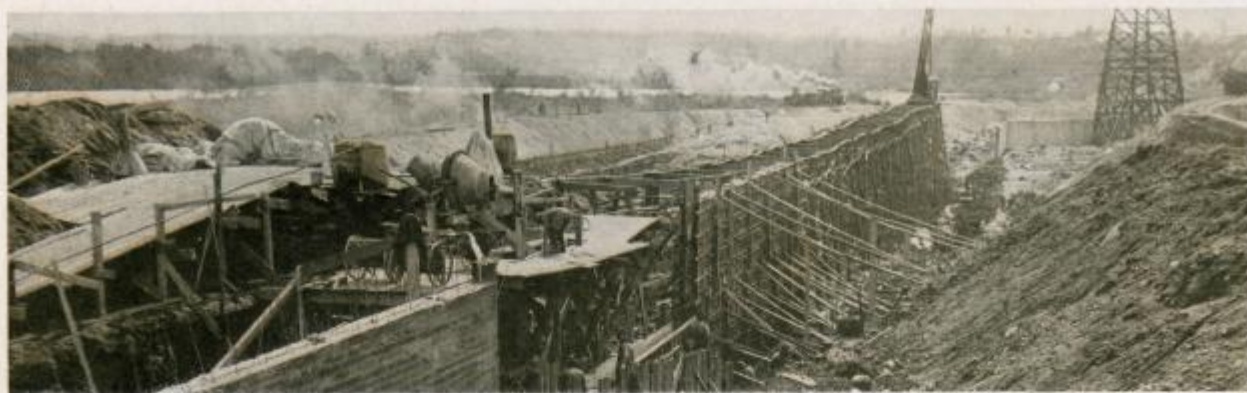
Pouring Concrete in Cofferdam
