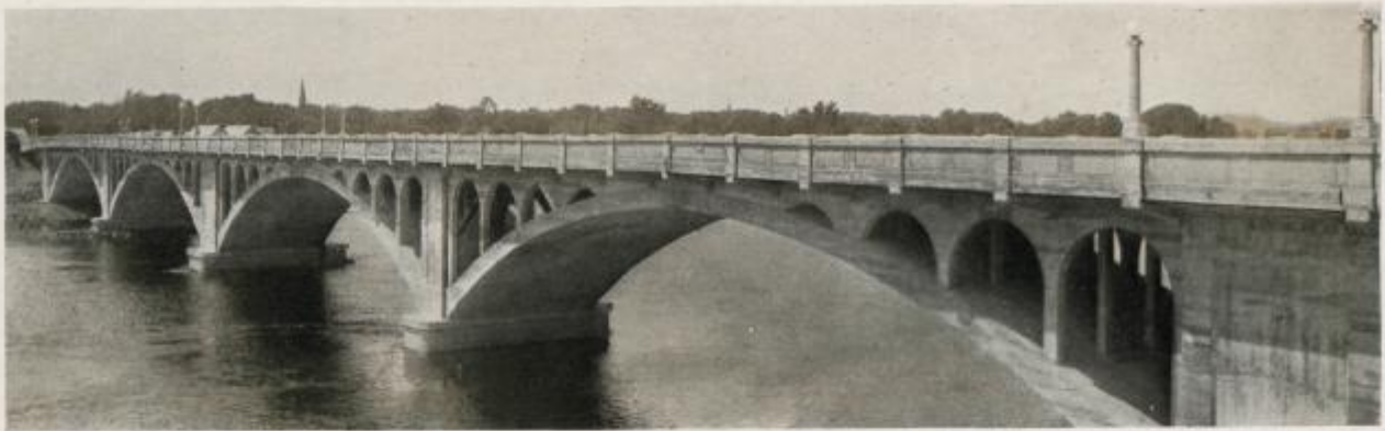
Concrete Bridge Over Chippewa River at Eau Claire, Wisconsin
