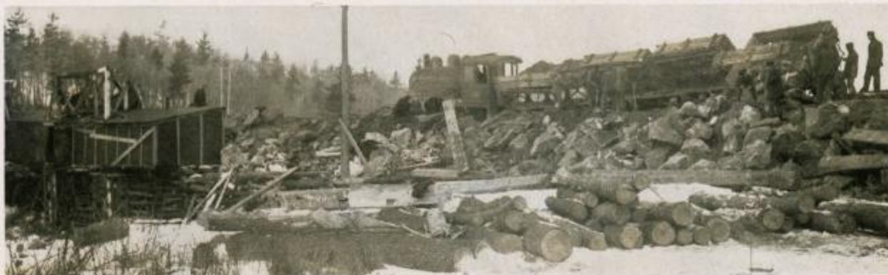
Completing Rock and Earth Embankment to raise lower Cofferdam
