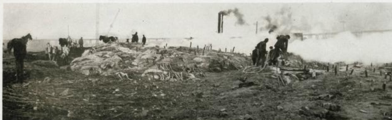
Excavating Rock in Spillway Channel
