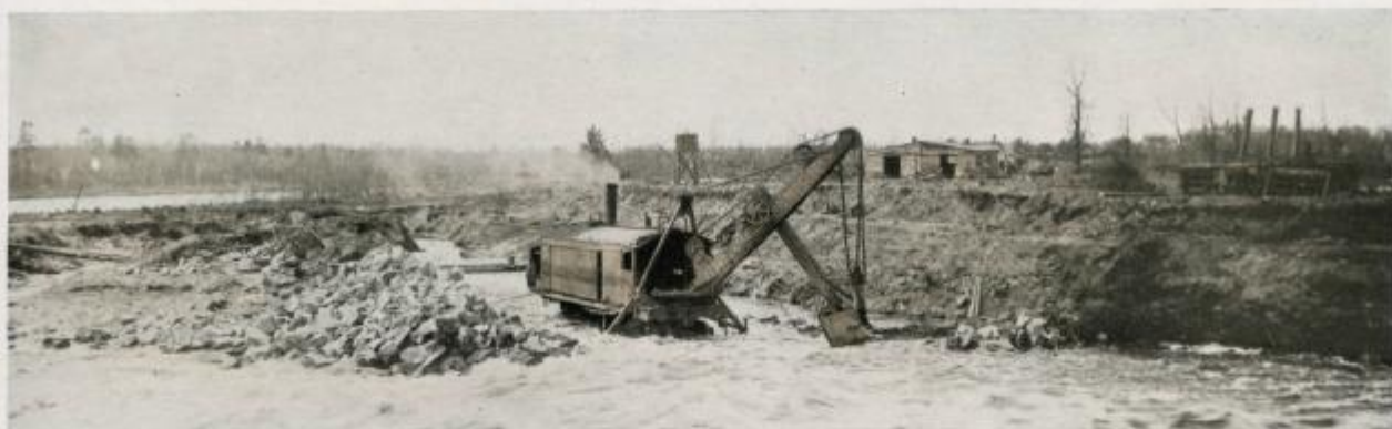
Shoveling Broken Rock From Foundations
