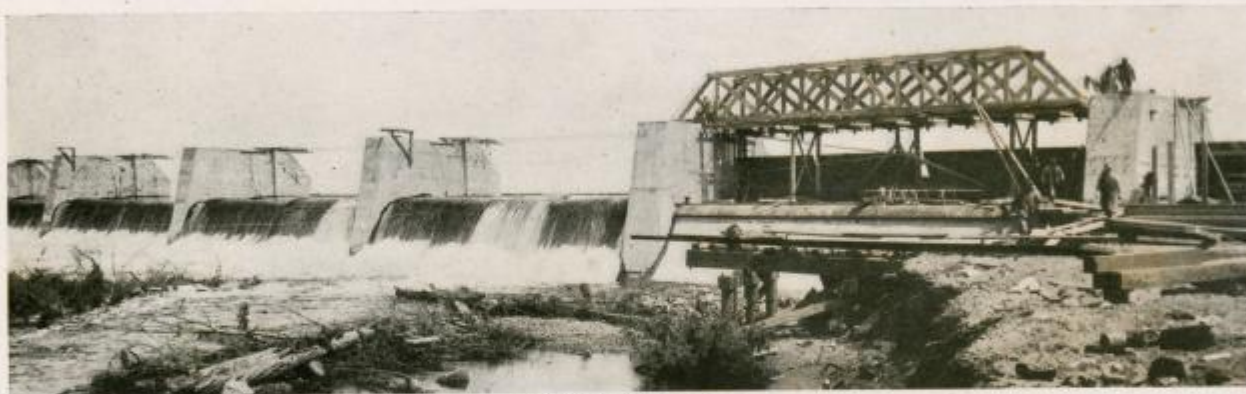
Placing Regulating Gates
