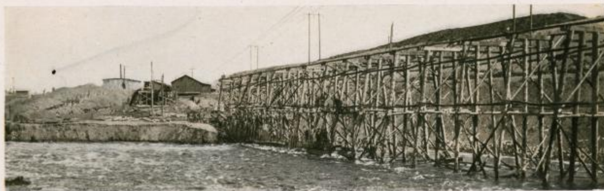
The Trestle for the Industrial railway
