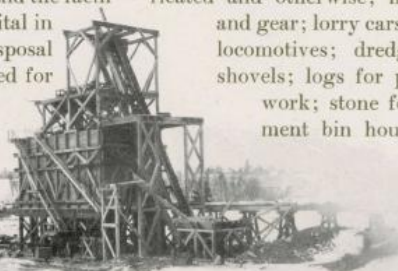
Gravel Washing Plant
