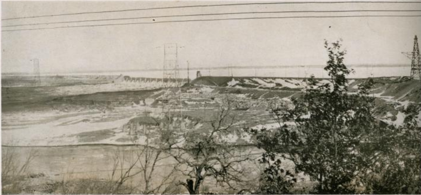
Down Stream View of Wisconsin Dam
