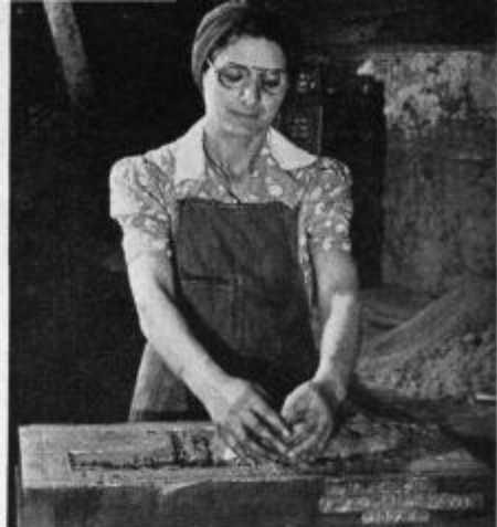
Coremakers have a big part in bringing tractors to life. Augustine Panosian is making cores for the pre-cleaner intake manifold of our Springfield crawler type tractors which are seeing action on world-wide battlefronts.
