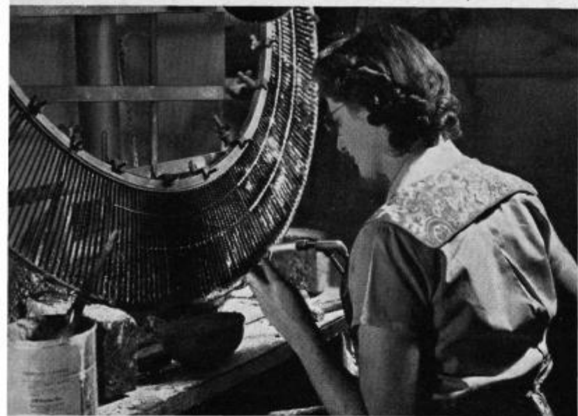
The steel blades in this jewel-like turbine ring were filed, polished, and set by girls. Marcella Gimler, West Allis, with silver solder and gas and air flame brazes each blade firmly into place.
