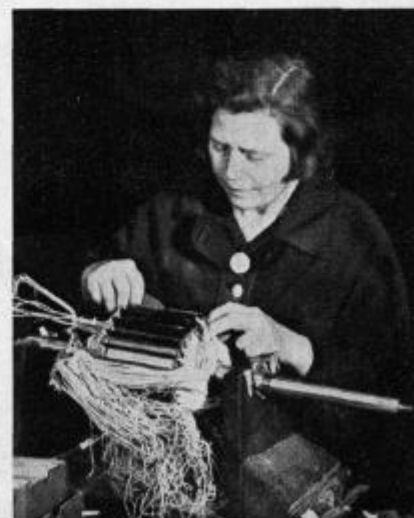
Hazel Moorman keeps scores of wires from crossing as she winds a small DC armature in our Norwood Works.
