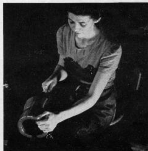
As her work-contribution to Victory, Violet Yurich, Pittsburgh, tapes a coil on a PD Current Transformer—a type of work women workers have been doing at Allis-Chalmers for more than forty years.
