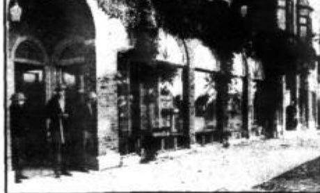
Recreation building, showing three deputies and Kohler show windows which were broken.
