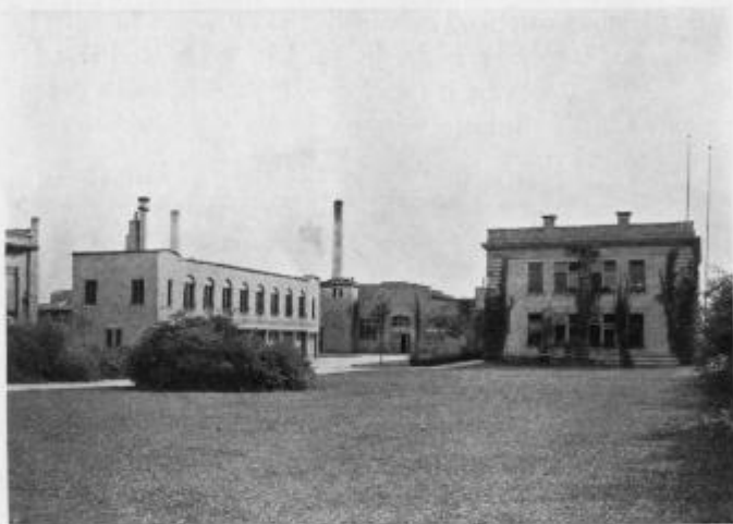
In the Vicinity of the Plant
