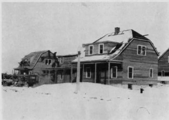
Homes Under Construction at Kohler
