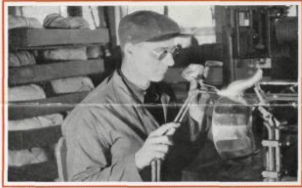
15 Welding on the spout. Mirro utensils are perfectly smooth, both inside and out.
