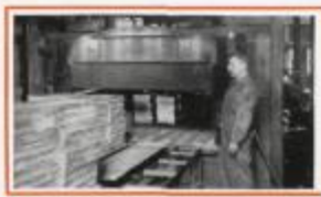
6 Slabs are then heated to high temperature preparatory to breaking down into plates.
