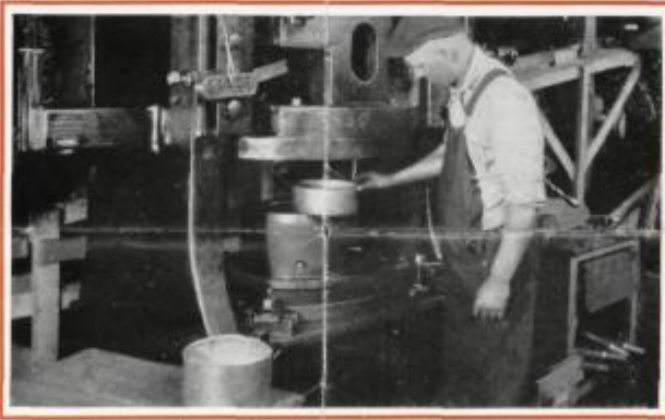
9 Cold stamping and drawing. Some Mirro utensils are given twelve draws to insure uniformity of thickness.
