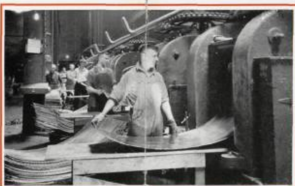
8 Plates are then cold-rolled into sheets. The farthest machine gives each sheet its hard, smooth Mirro surface.
