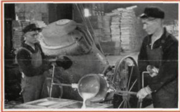
5 After leaving the heating furnace, the pure aluminum is cast into fifty pound slabs.
