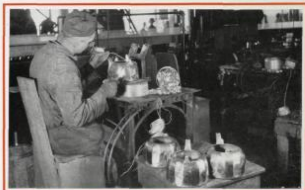
14 Welding on the ears. No rivets or clinching in Mirro—no dirt-catching crevices.
