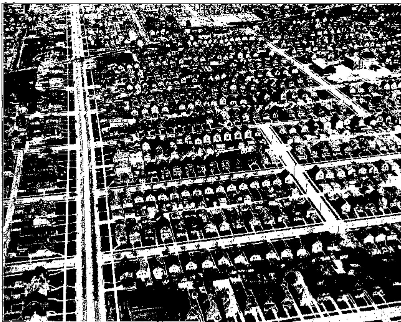
In the Northwestern Section of Milwaukee, Showing Capital Drive, which extends from the Shore of Lake Michigan to Madison, a distance of 95 Miles
