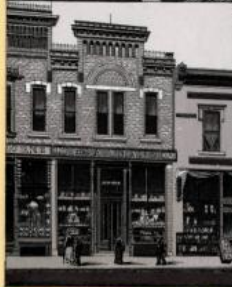
JAS. A. TRANE PLUMBING HOUSE.
