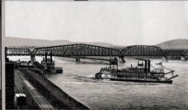
NEW MISSISSIPPI RIVER WAGON BRIDGE.
