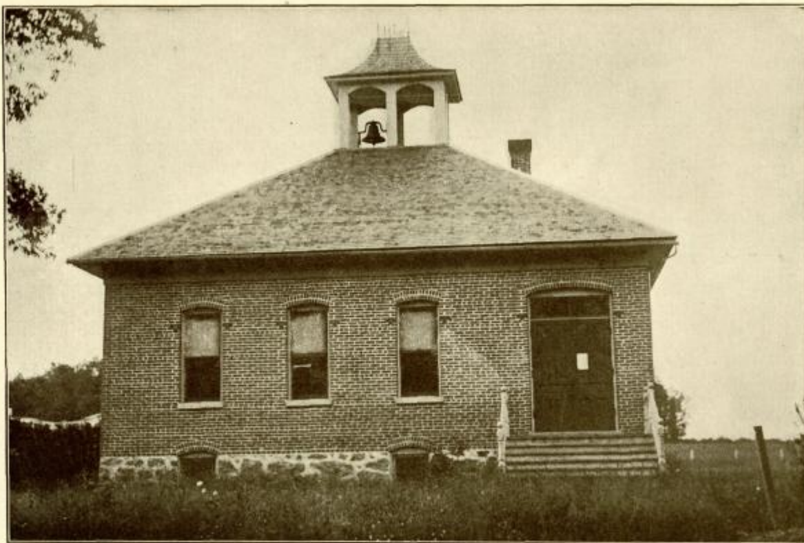
ONE OF THE MODERN RURAL SCHOOL BUILDINGS IN WISCONSIN. District No. 3, Town of Amherst, Portage County.
