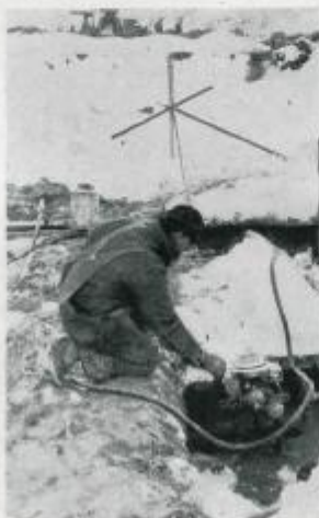
Supplying the Paver with Water
