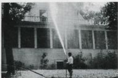
Nozzle at End of 200 ft. Hose Gives 20 ft. Elevation
