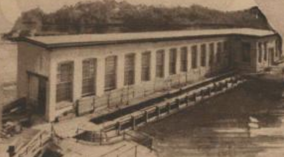
VULCAN POWER HOUSE APPLETON, WIS. Built 1909 Developing 30,000 K. W. H. per day, most of which is transmitted electrically to Kimberly
